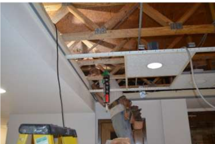
The work was sometimes in tight, hard to reach spaces.
