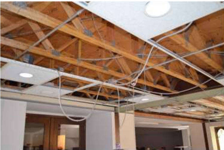
Exposed trusses before reinforcement.
