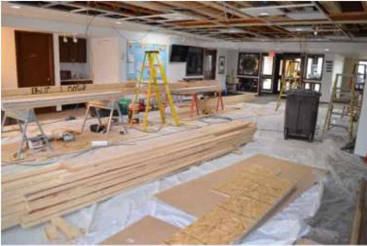
Narthex during construction.
