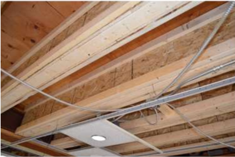
Finished reinforced beams.
