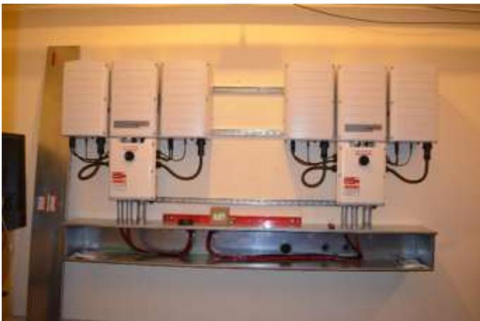
The Power Inverters are in place and ready for Final wiring.
