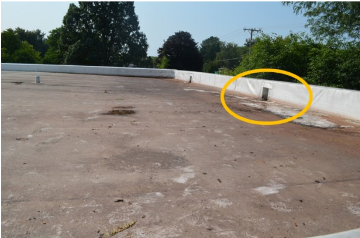
Drained Roof – One of the roof drains is circled
